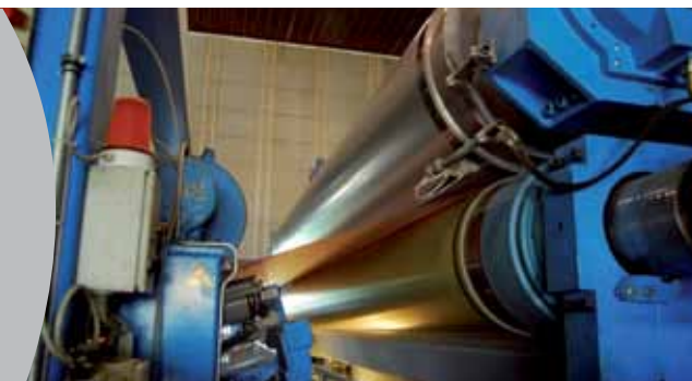
HOT ROLLING MILL
